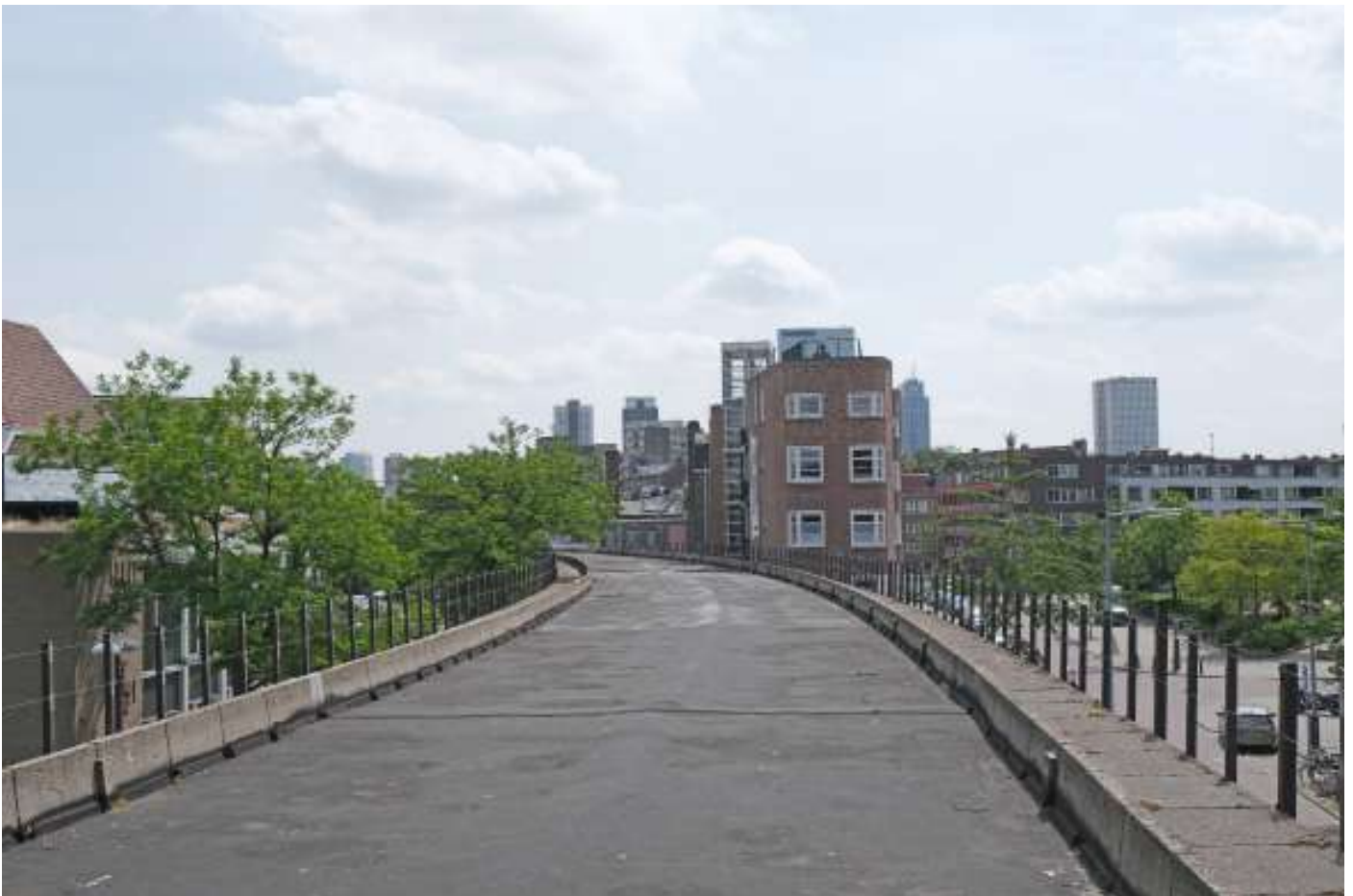
25 Current situation: roof view in the Northern part. Spoorpunt
