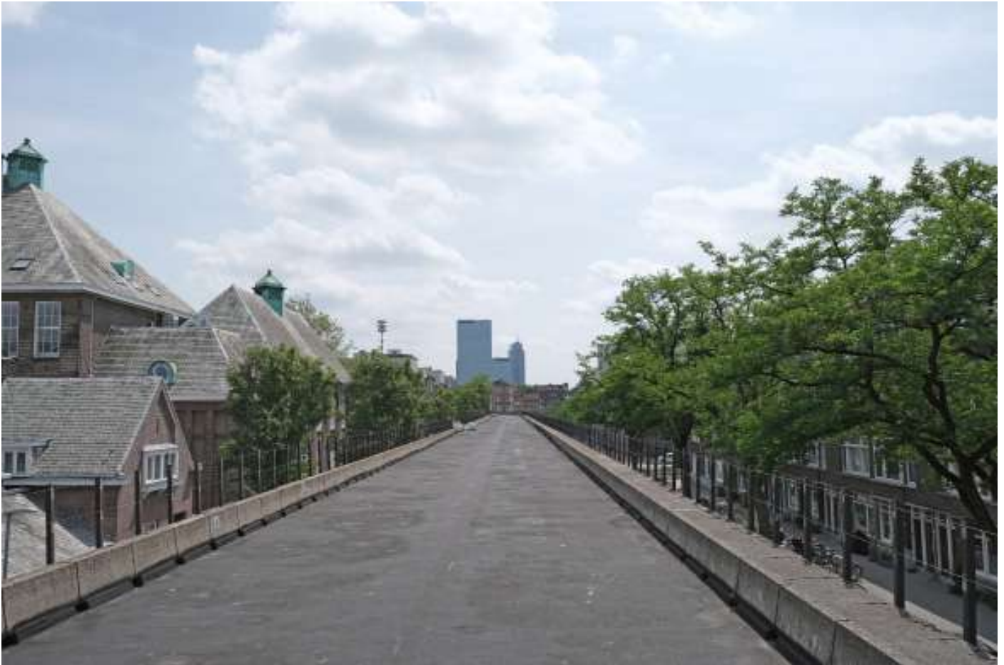
24 Current situation: roof view - Bergpolder towards city centre
