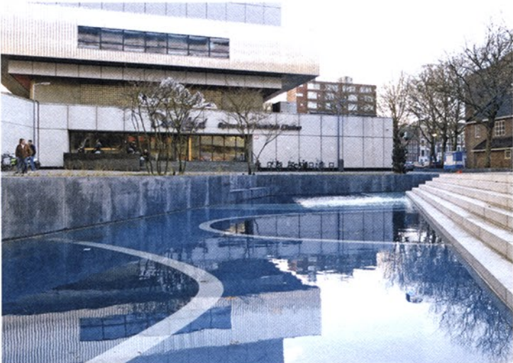
About 15 times a year the excess runoff will flow onto the square.
