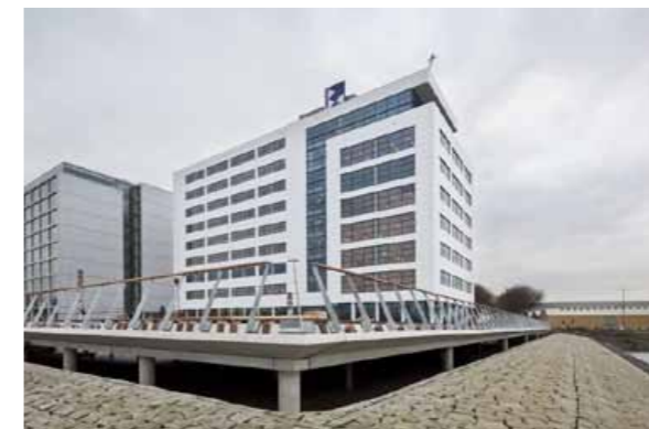
Port City Rotterdam, wet-proof construction
