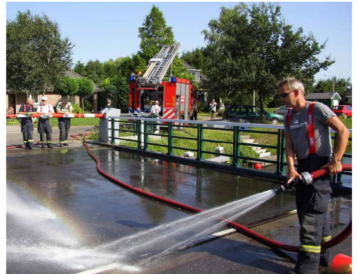
Spraying a bridge with water to prevent malfunctioning due to heat expansion
