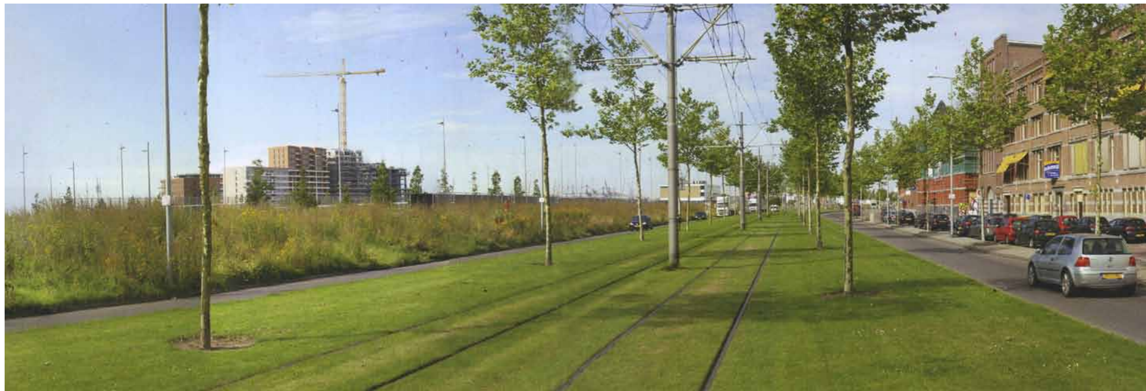
The primary dikes form an attractive green landscape with elevated cycle path along the Westzeedijk
