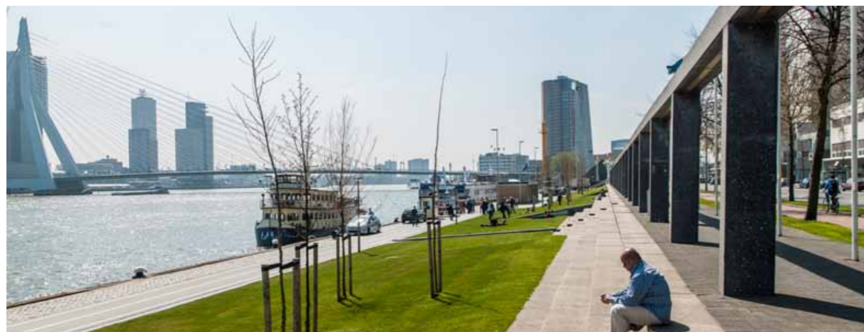
The primary dikes along the recently renovated Boompjes form an attractive recreational landscape by the river Meuse
