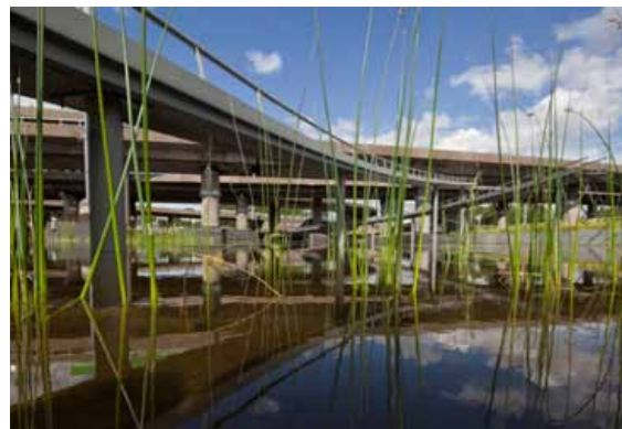
Temporary water storage under the Kleinpolderplein motorway interchange
