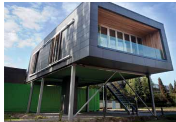
Concept House Village Heijlplaat, flood-proof construction
