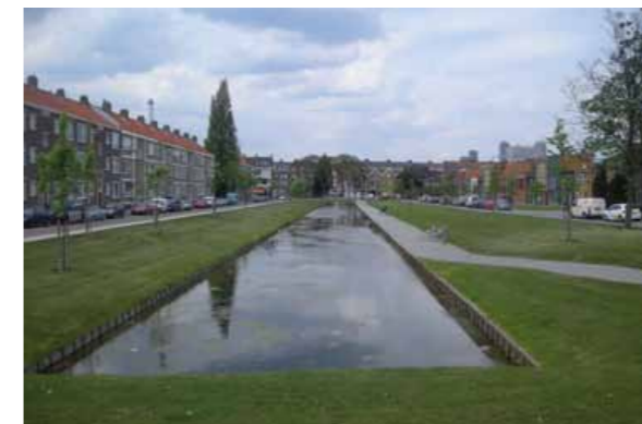
Extra surface water in the form of a new canal
