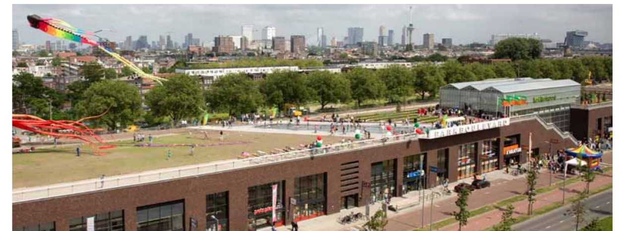
The roof top park Vierhavenstrip is a public outdoor area in a unique, multi-functional dike setting
